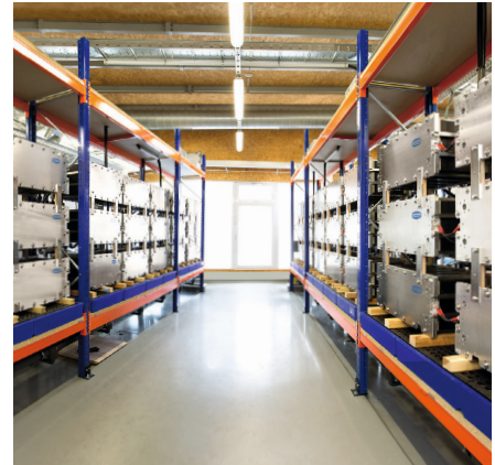
The redox-flow large-battery storage facility at the Fraunhofer ICT in Pfinztal: the pilot system is equipped with Schmalz Stacks.
