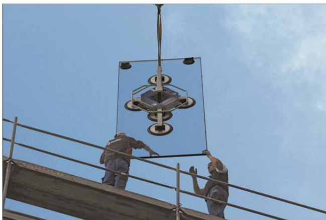
VacuMaster Glass being used for outdoor glass handling
